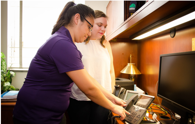
ITCS student employees assisted staff with upgrading VoIP phones across campus as part of an extensive modernization project.
